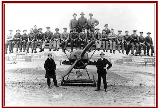
289. This photograph how simple the wings have been assembled on threstles only.
